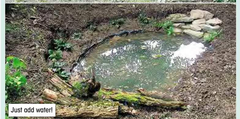
Once you are happy with the shape of your pond, install the underlay, the liner and the plants.
