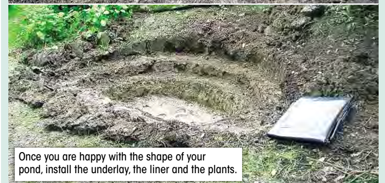
When digging a new pond, make sure to include ledges on which to plant marginal species.
